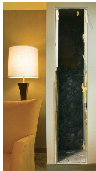
Remove internal components and trim cabinet edges.
