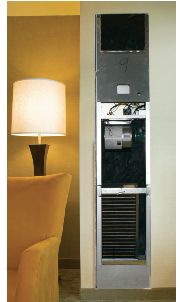
Remove surface components and trim drywall.
